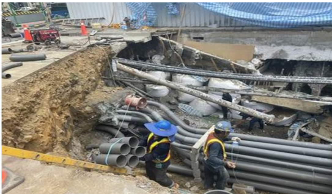
Figure 10. Exposed pipelines under a road.
