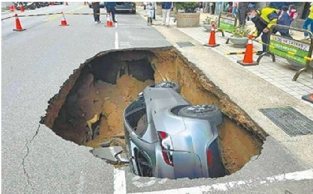
(b) The second road sinkhole
